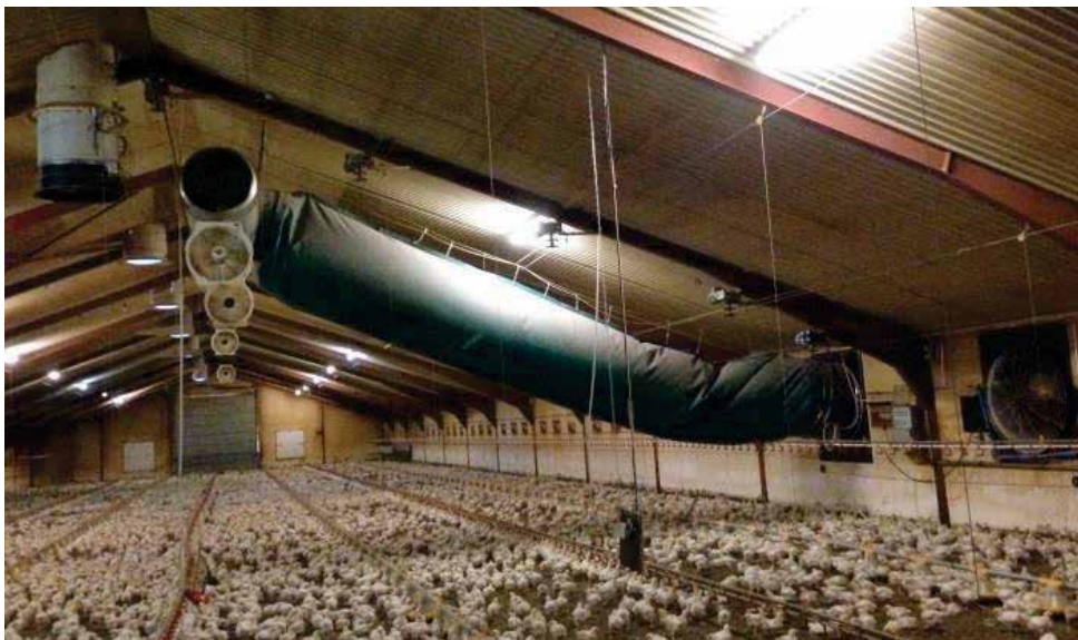
Figure 2 (A and B). The Agro Clima Unit situated outside a broiler house (A). Ventilation air to and from the broiler house are drawn through the Agro Clima Unit by a countercurrent principle to utilize the heat content of out flowing air to heat up inflowing air. Figure 2 B shows the tube transporting the heated air to the ridge of the broiler house in test farm 1.
